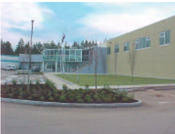
Oceanside Place Multiplex Arena
