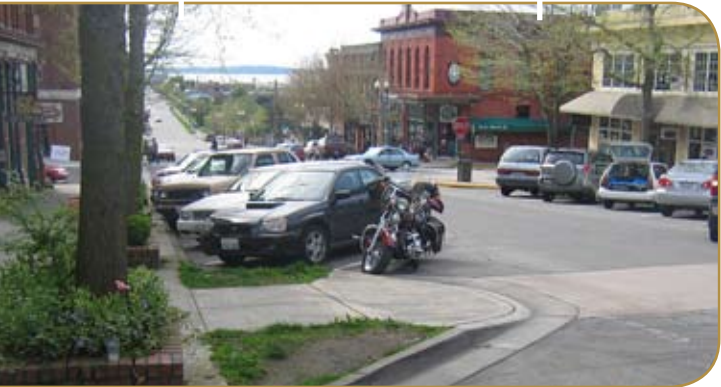
At street corners, bulges can control the flow of traffic and increase safety for pedestrians as they decrease exposure to car traffic by reducing the distance from curb to curb and improve pedestrian site lines/ visibility
